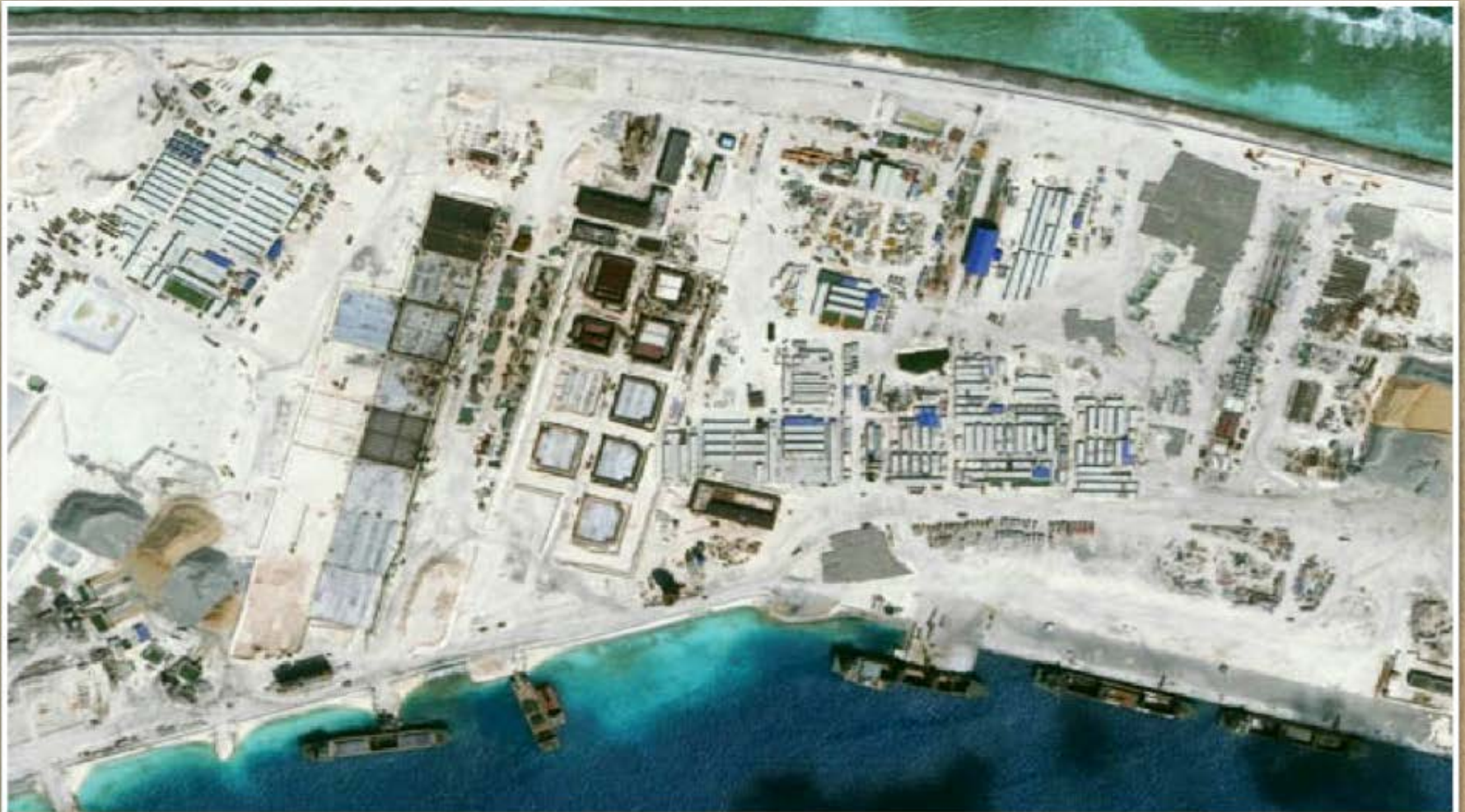
The northwest side of Mischief Reef as of January 8, including a 1,900 foot seawall and newly-constructed infrastructure including housing, an artificial turf parade grounds, cement plants, and docking facilities.
