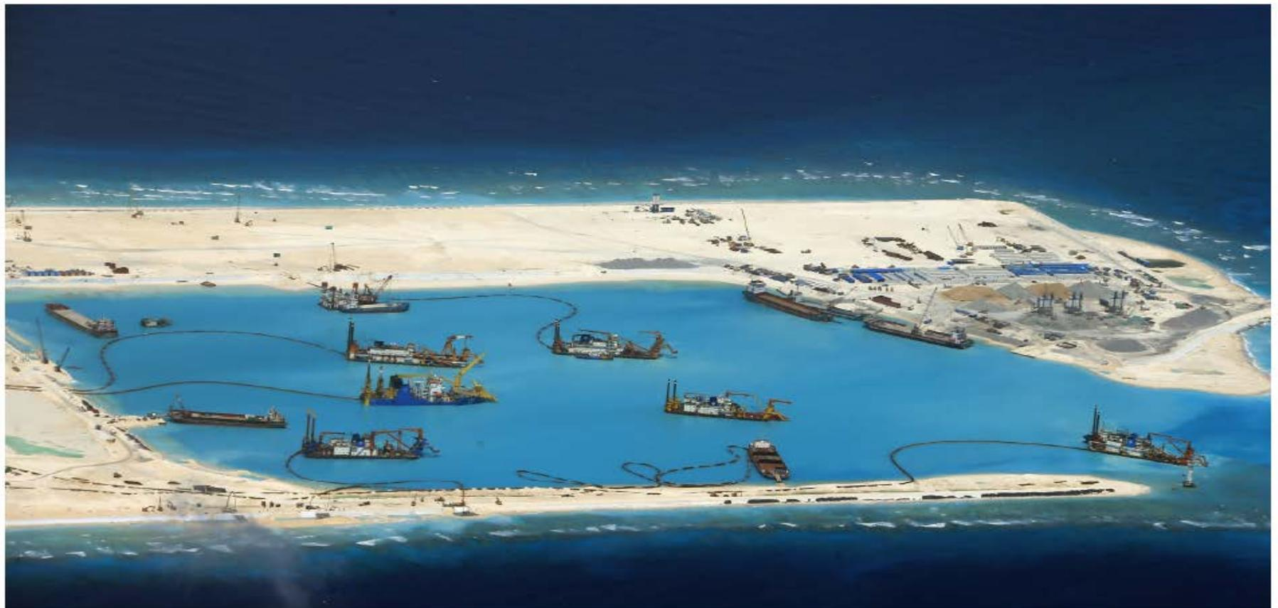
**Seven (7) cutter suction dredgers and seven (7) cargo/supply vessels
